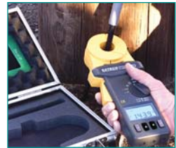
Verify resistance of cellular and communication tower ground grids
