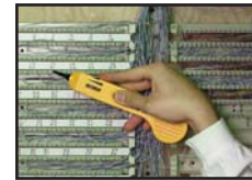
Trace phone/data wiring
