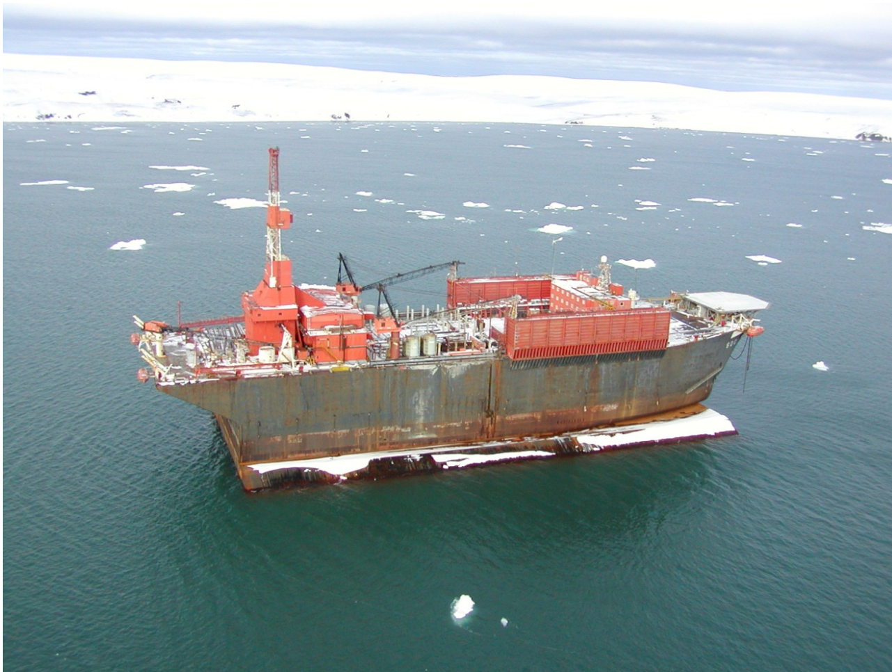
Figure 15. The Steel Drilling Caisson (SDC).
