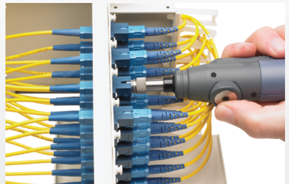
Patch panel bulkhead inspection
