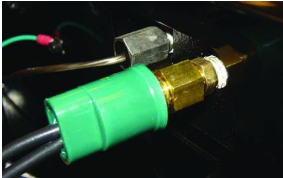
Figure 5.13 Pressure Switch and Schraeder Adapter
