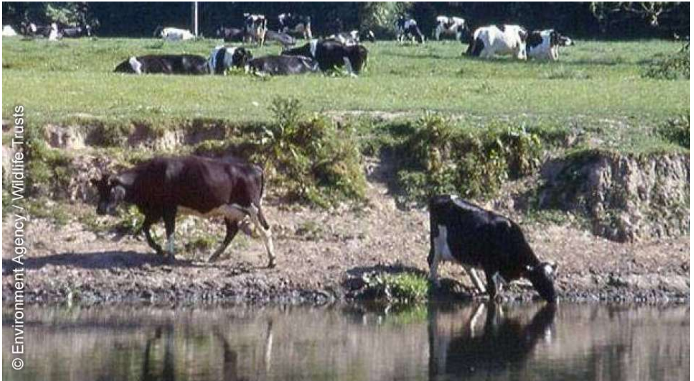
Figure 13. Bank failure can occur due to over-stocking.
