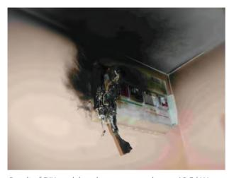
Result of DIY work by a home owner where a 10.5 kW electric shower was connected to a 45 A circuit-breaker using 2.5 mm<sup>2</sup> cable. (Photo courtesy of British Gas)
