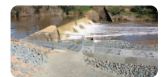
Fishways allow fish to move around barriers such as weirs (JO)
