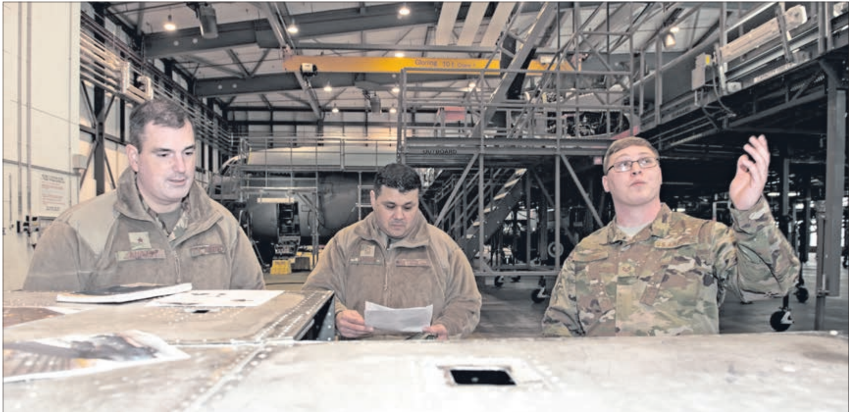
U.S. Air Force Staff Sgt. Justin Cupit, 86th Maintenance Group facility manager (right), discusses plans to install a fall prevention system with U.S. Air Force Brig. Gen. Mark R. August, 86th Airlift Wing commander (left), and U.S. Air Force Chief Master Sgt. Ernesto Rendon, 86th AW command chief (middle), in the dual bay hanger on Ramstein Air Base, Jan. 24. August awarded Cupit as the Airlifter of the Week for his efforts in maintaining more than 40 86th MXG buildings worth more than $60 million.
