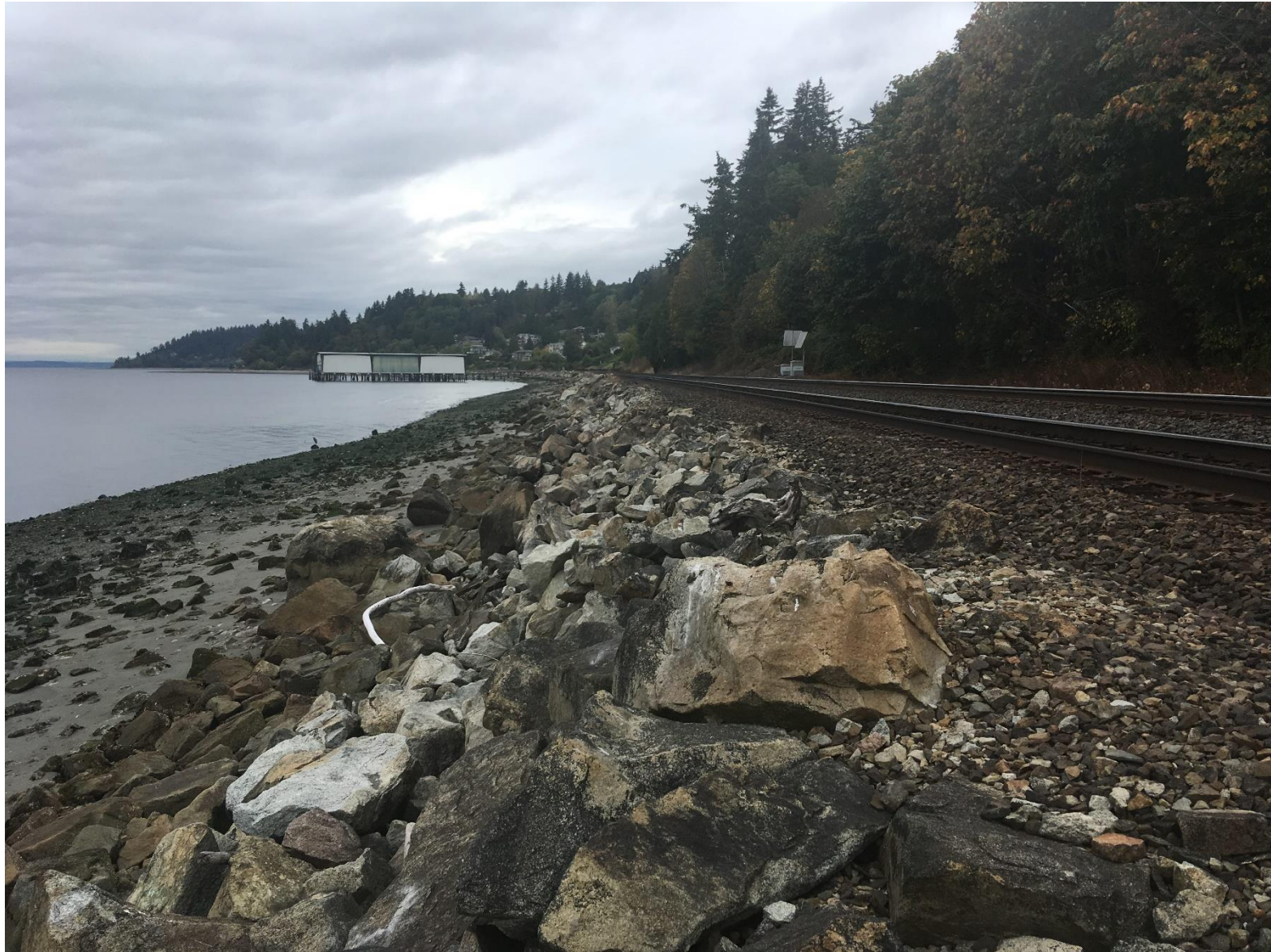
H-9: View of shoreline looking north, 2018.
