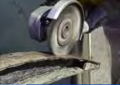
Prepping a machine guard for on-site welding and repair.
