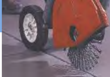
Cleaning a crack on an airport runway prior to filling.
