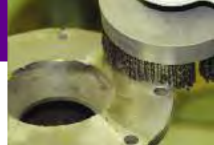
Removing gasket material from a pipe flange.
