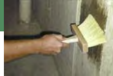
Applying waterproofing material with a masonry brush.
