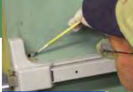
Painting a tight area on a steel door with a Marking Brush.
