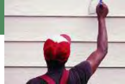
Applying paint to clap board siding.
