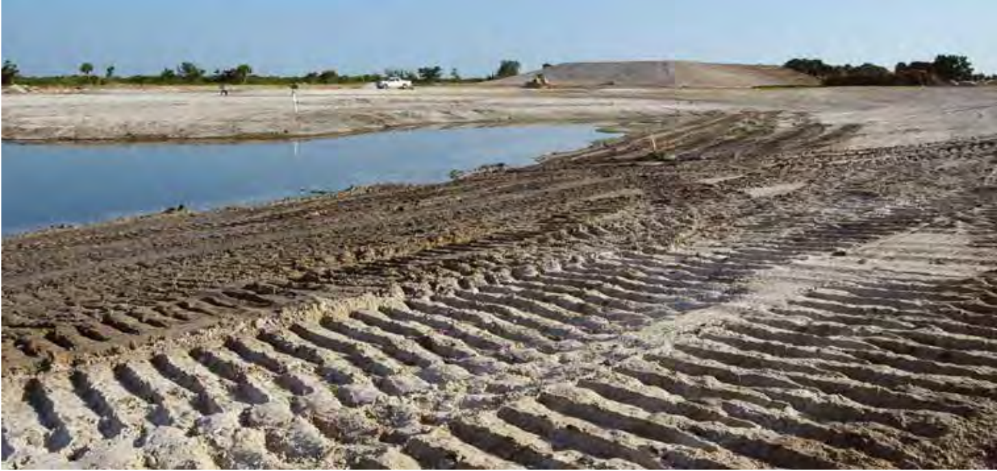
Construction on a lake shoreline. Greg Workman/FWC.
