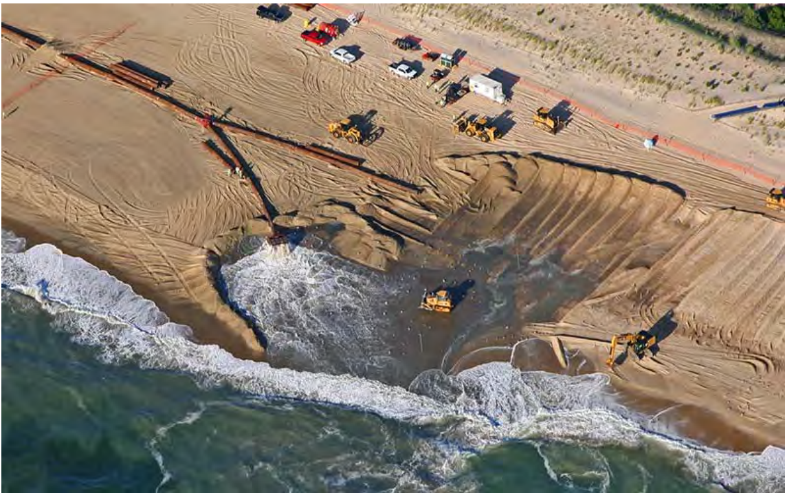
Figure 3-3. A Typical Beachfill Operation along the Delaware Atlantic Coast. (Source: Great Lakes Dredge and Dock Company website accessed at: http://www.gldd.com/company/projects/coastal-protection/ on 5/7/2015)
