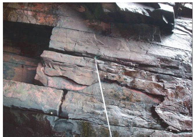
IMG0974.JPG Close up of piton, no fix possible.
