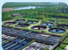
Water Treatment Plant System
