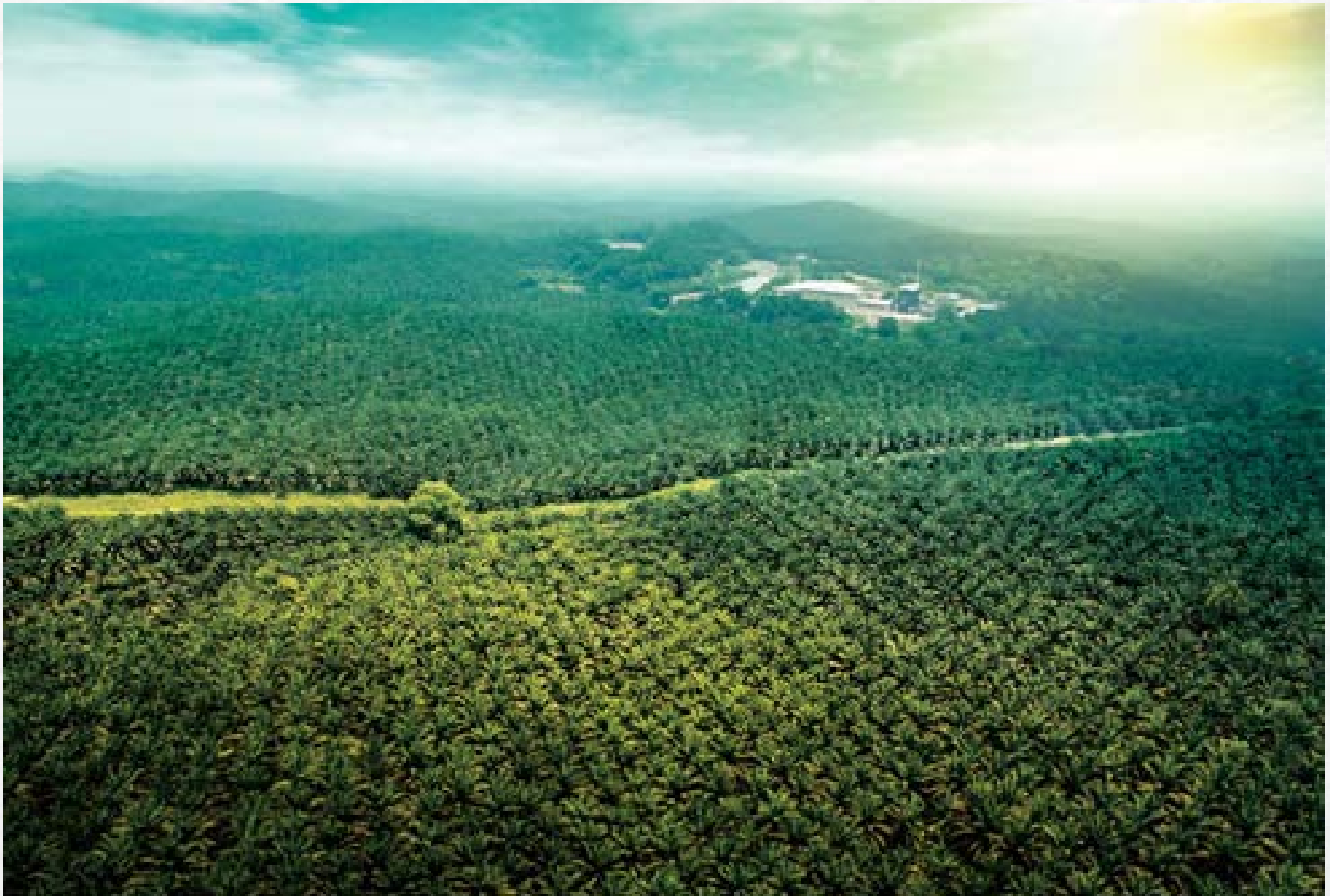
Jengka Biomass Power Plant, Pahang.
