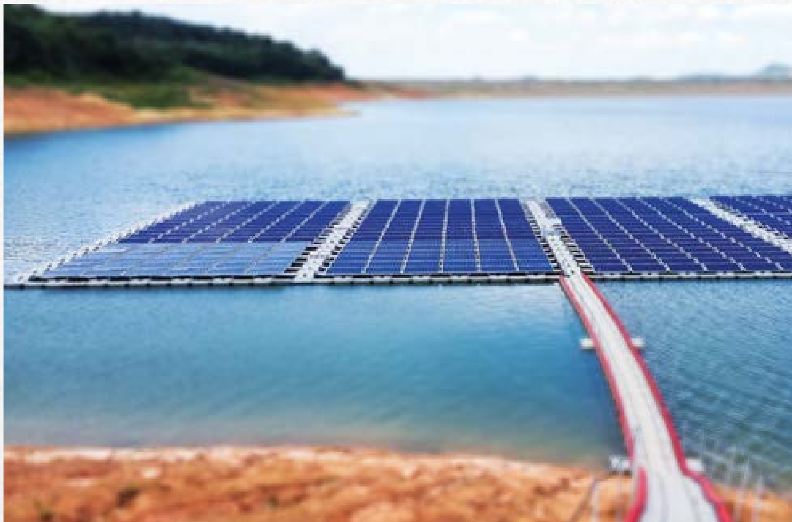
Floating Solar Photovoltaic System at the Sungai Labu Water Treatment Plant, Salak Tinggi Reservoir, Selangor.
