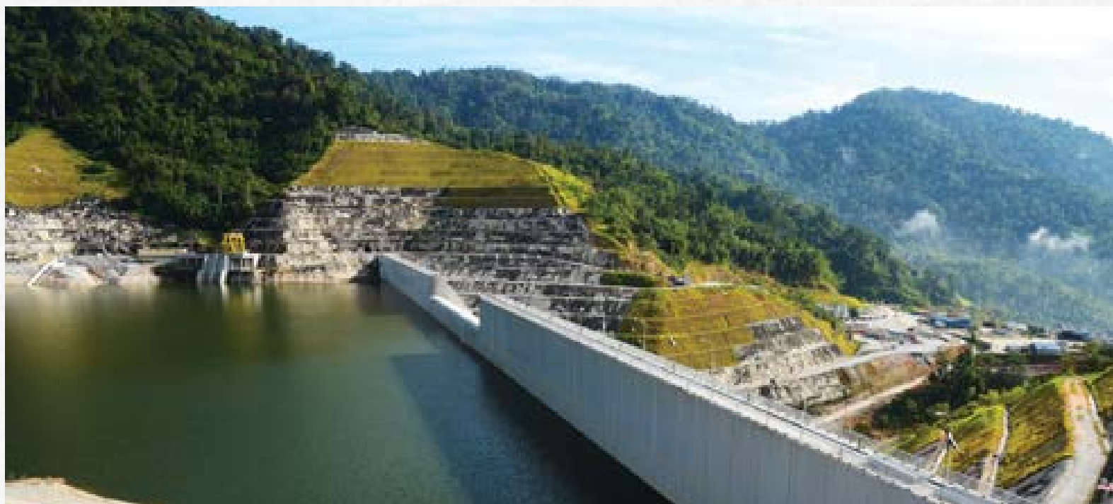
Ulu Jelai Hydroelectric Project, Cameron Highlands, Pahang.
