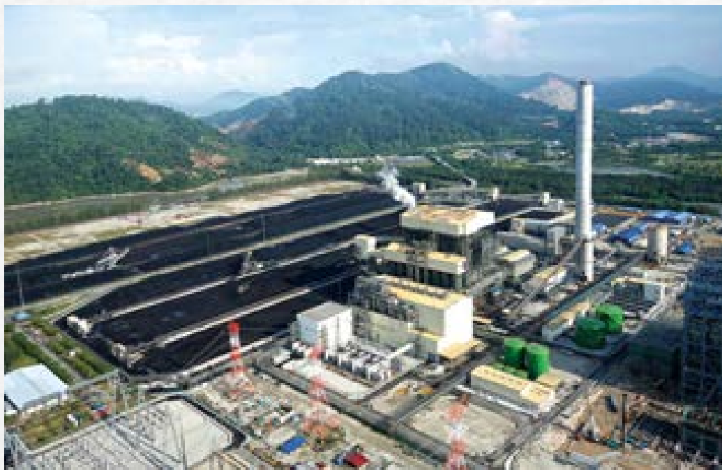
An aerial view of Manjung 4, Sultan Azlan Shah Power Station, Manjung, Perak.
