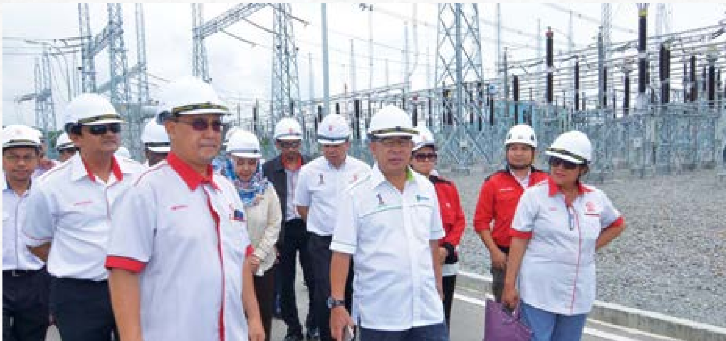
Minister of Energy, Green Technology and Water, Datuk Seri Panglima Dr. Maximus Johnity Ongkili during the launch of Kimanis Main Intake Substation in Papar, Sabah.
