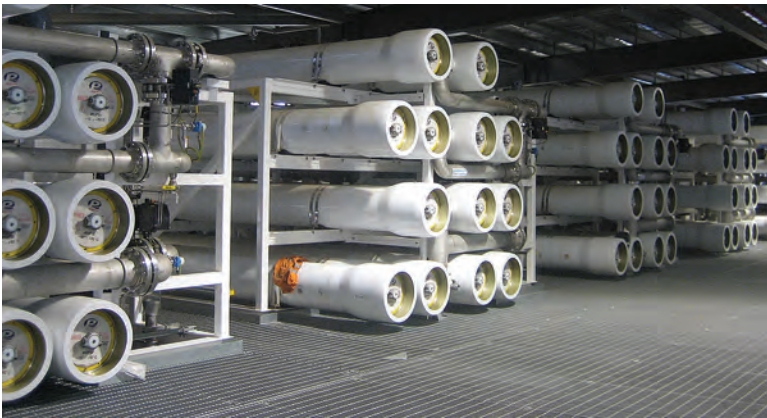
Some equalization ahead of the RO is usually needed to simplify operation, reduce operation and maintenance costs, and maximize production of reclaimed water.
