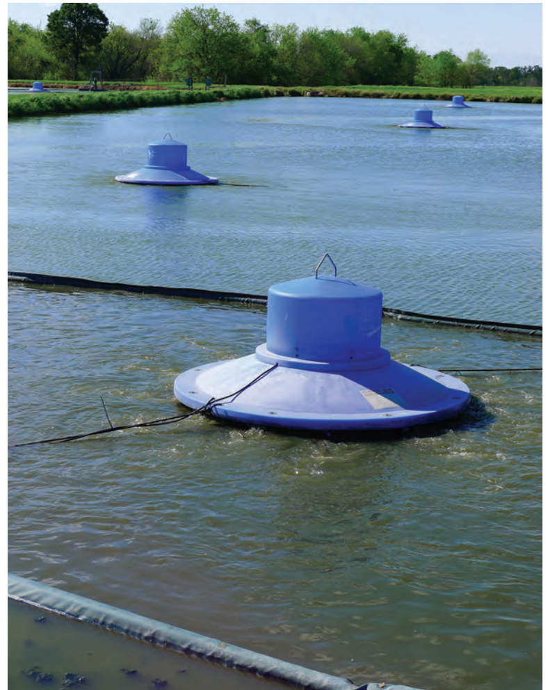
An aerator with a specialized engineered biofilm is used for ammonia reduction.
