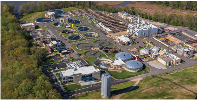
The 24 mgd H.L. Mooney Advanced Water Reclamation Facility serves 250,000 customers in and around Woodbridge, Virginia.
