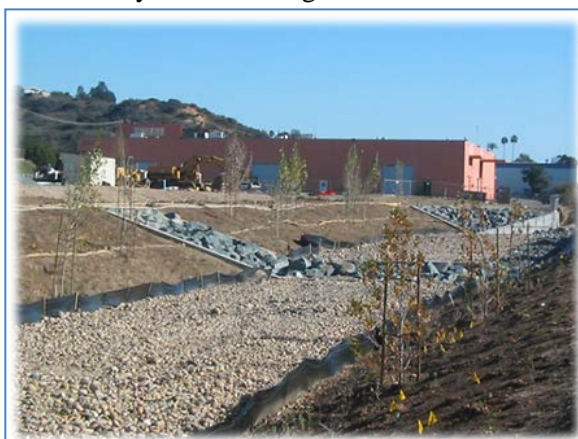
In-Line Stream Restoration Project – Increase Channel Capacity and Floodplain to Create More Stable System
