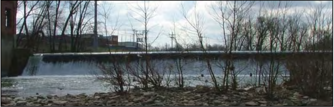
Photo 17: The Shelbyville dam, Duck River, TN.
