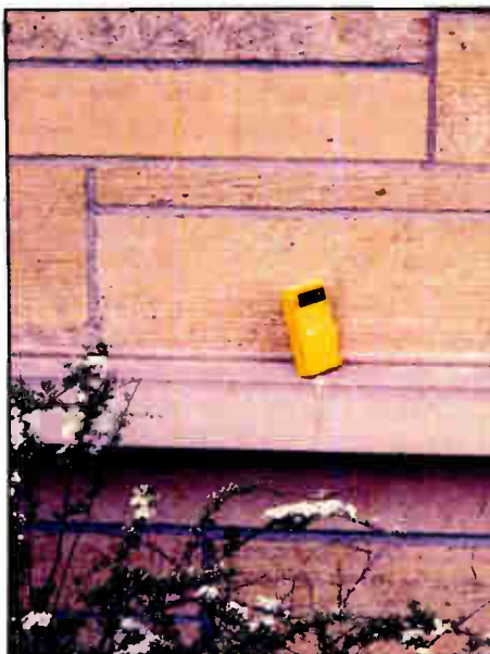
Transponder in place.
