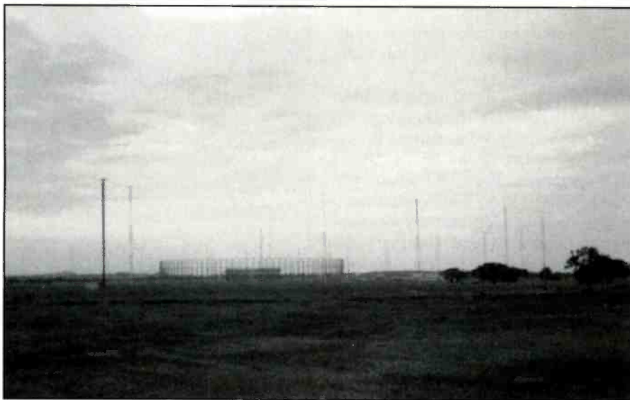
The circular antenna array is a FLR-9 which was used by the 6922nd Electronic Security Squadron at Clark Field, Phillipines. The other antennas are suspected of being the receiving antennas for KWL90, U.S. Embassy, Manila. Photo was taken in 1990 by Tom Severt, KS.
